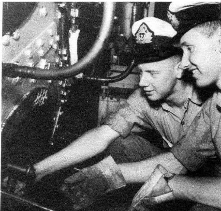
Cadet George Bot Explains Changing Routine of Oil Sprayers in One of Ontario's Boiler-rooms to Cadet Art Griffin.
